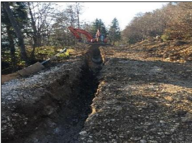
St-Brais-Sceut. Interconnexion eau potable des 2 villages.
