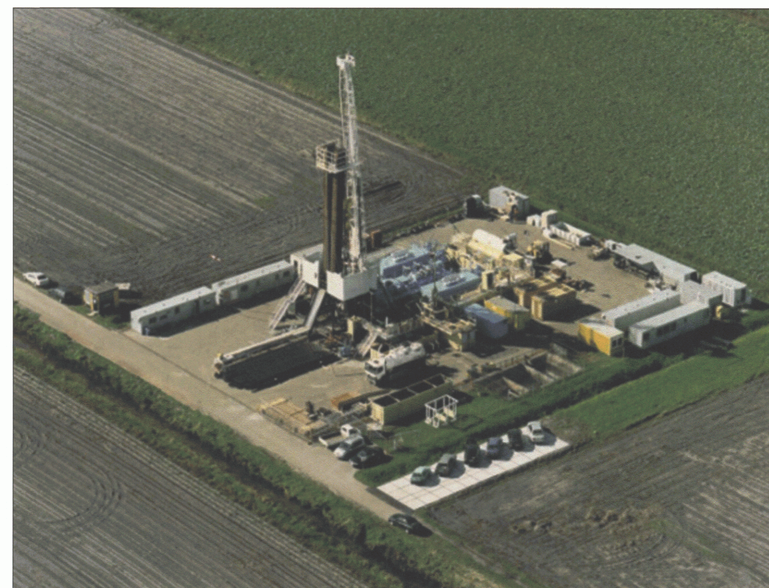
Installation de forage
