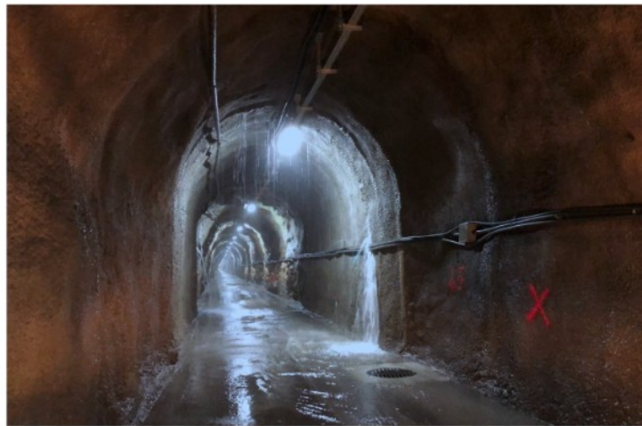
Figure 2: HS: Significant water inflow into the Safety Gallery at the base of the St-Ursanne Formation (Photo: S. Schefer, swisstopo).
